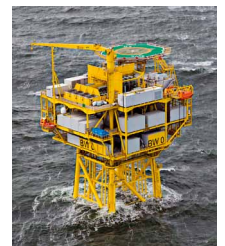
Borkum West II Substation Platform German North Sea
