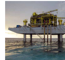
SANAGA 01 gas MOPU
