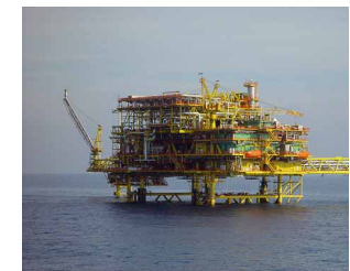
Bunga Raya - E Gas Treatment Platform
