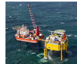
MOAB® AC Substation for GLOBAL TECH 1 Wind Park German North Sea
