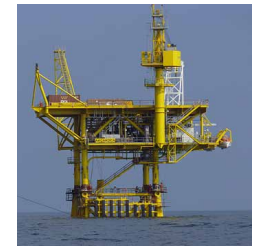
AKCAKOCA Gas Wellhead Platform
